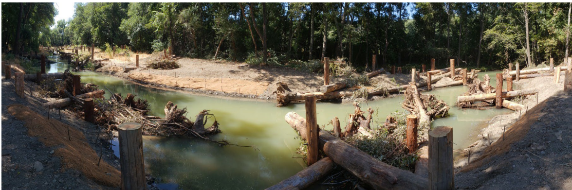
Photograph of the completed 13B inlet project. Photograph showing the newly constructed habitat features at the inlet to the 13B side-channel. The area in the far upper-left of the side-channel is the portion construction in 2022.
