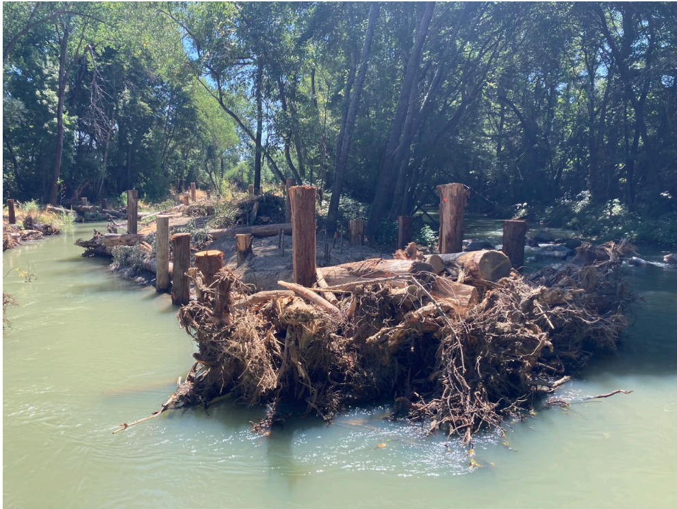
Photograph taken on August 8, 2023 of the completed 13B inlet project. The photo is showing an apex logjam structure at the inlet with the mainstem flow of Dry Creek to the right of the log structure and flow on the left entering the constructed side channel habitat feature.
